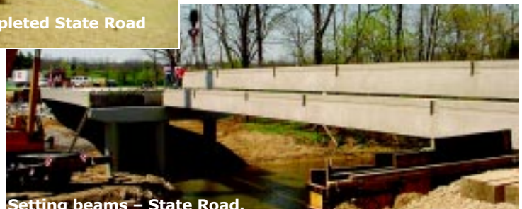
Setting beams – State Road.
