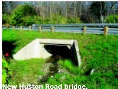
New Huston Road bridge.
