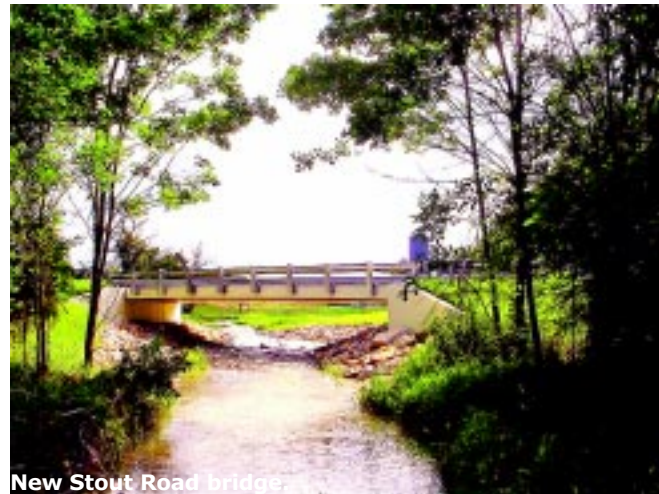
New Stout Road bridge.
