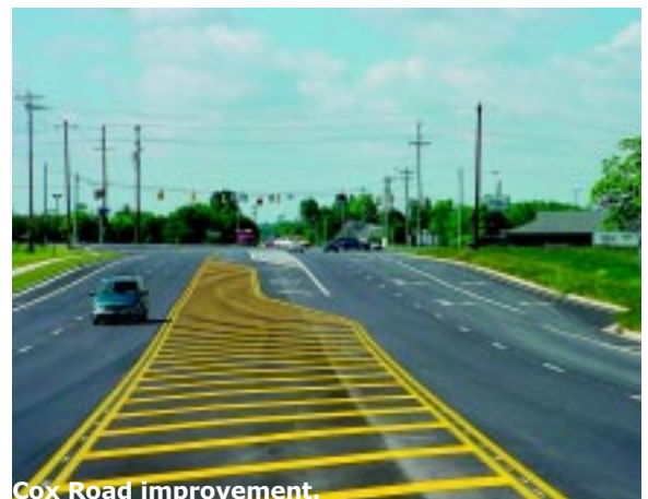
Cox Road improvement.
