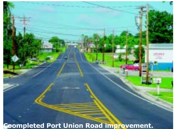
Completed Port Union Road improvement.
