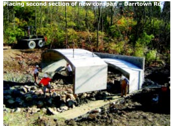
Placing second section of new conspan – Dartrtown Rd
