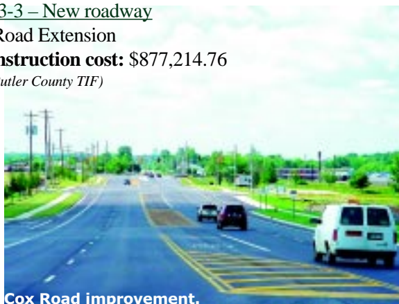
Cox Road improvement.
