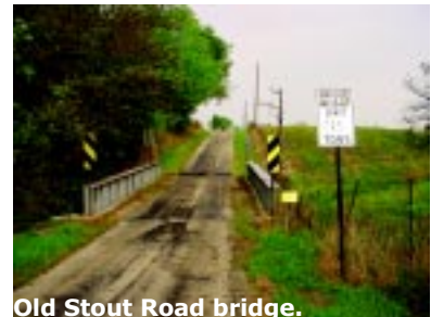
Old Stout Road bridge.
