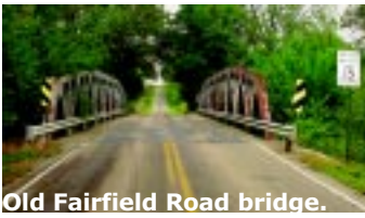
Old Fairfield Road bridge.
