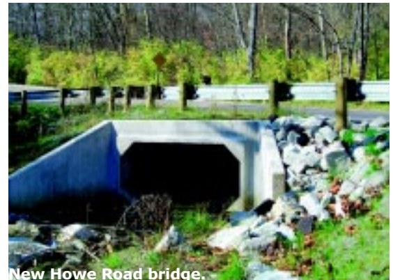
New Howe Road bridge.
