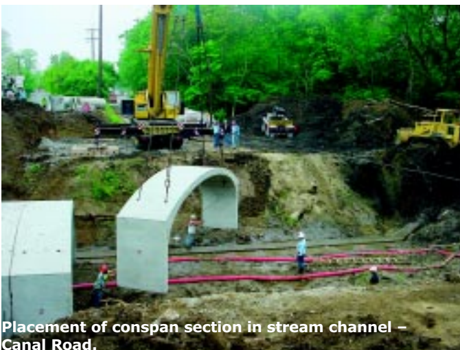
New conspan in place – Canal Road.
