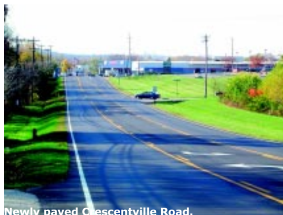
Newly paved Crescentville Road.
