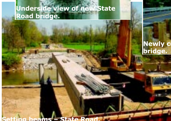
Setting beams – State Road.
