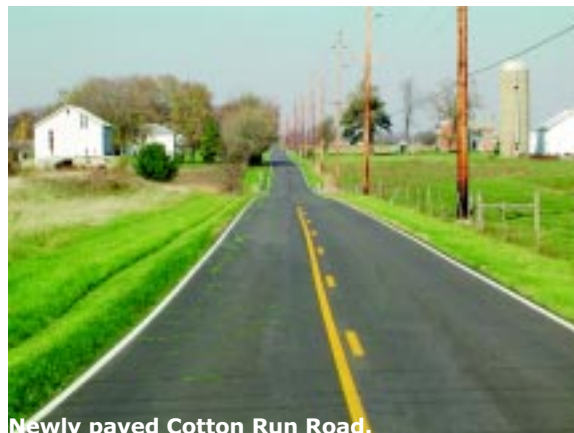
Newly paved Cotton Run Road.
