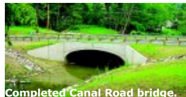
Completed Canal Road bridge.
