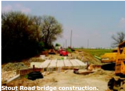
Stout Road bridge construction.
