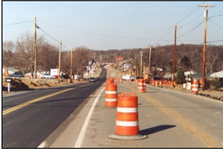
Cincinnati Dayton Road will be widened to five lanes.
