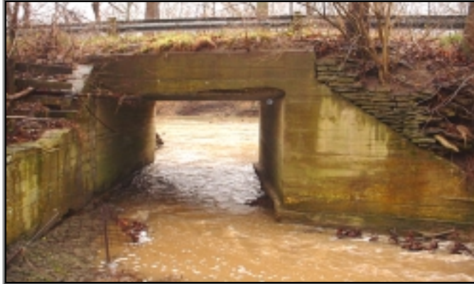
Existing Four Mile Creek Road Bridge #01.870.
