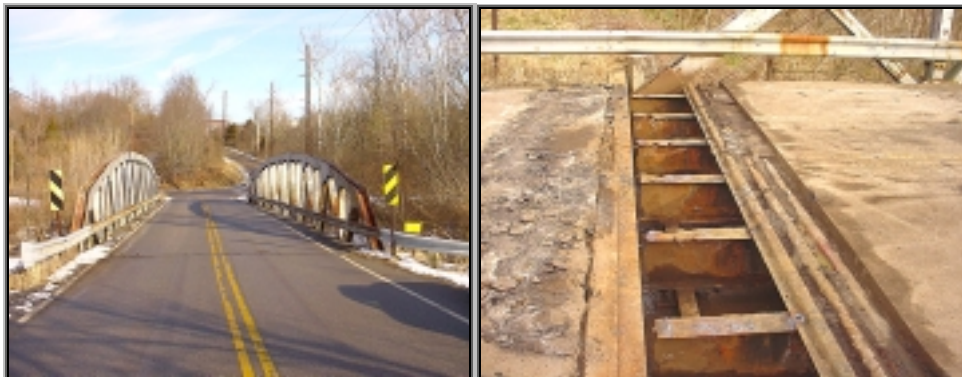
Indian Creek Road Bridge #01.360.
