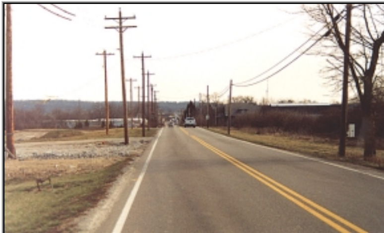
Port Union Road view east. The road will be widened to three lanes – one in each direction plus a center turn lane.
