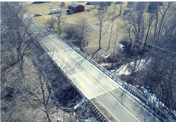
TOLBERT ROAD SUPERSTRUCTURE #0.914 Superstructure Replacement Total Construction Cost: $440,114.00 Funding: BCEO
